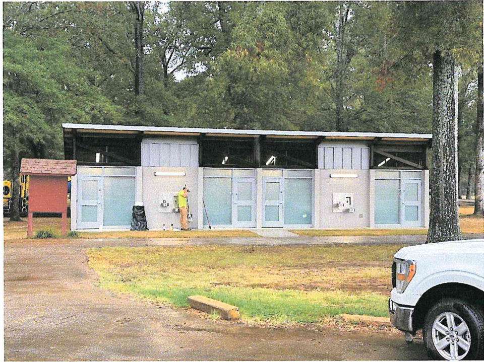
Figure 1 – Roger's Park restrooms complete
