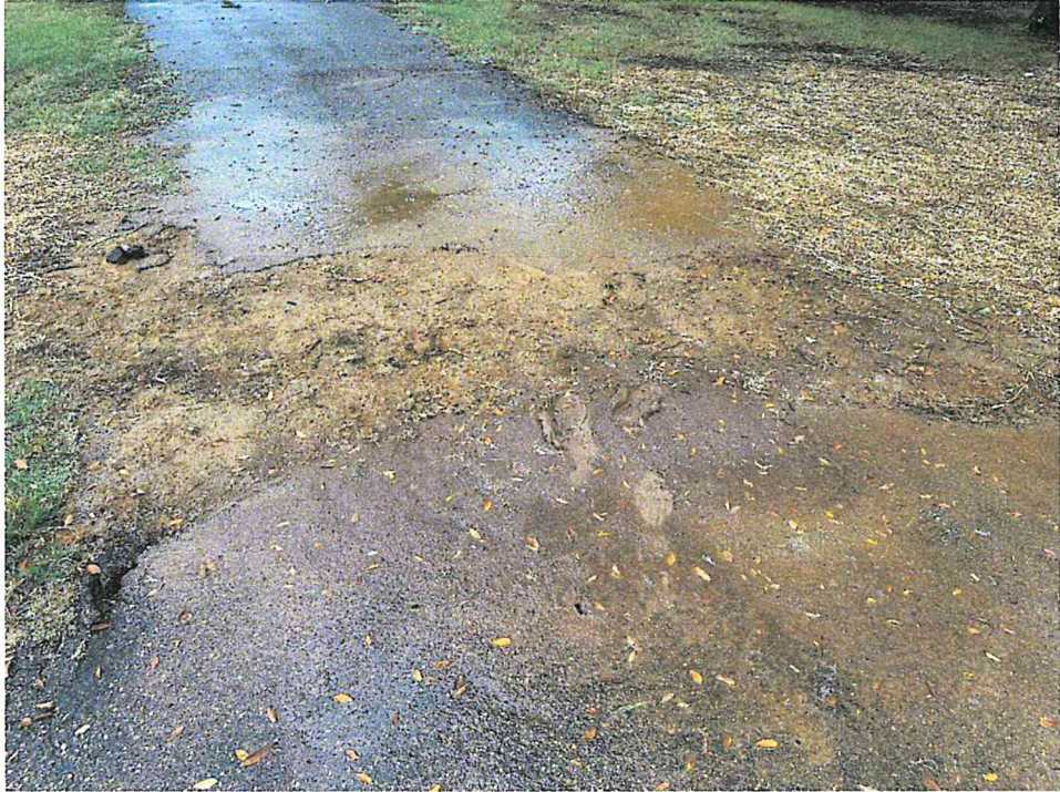
Figure 7 – Repair track where new piping was laid.
