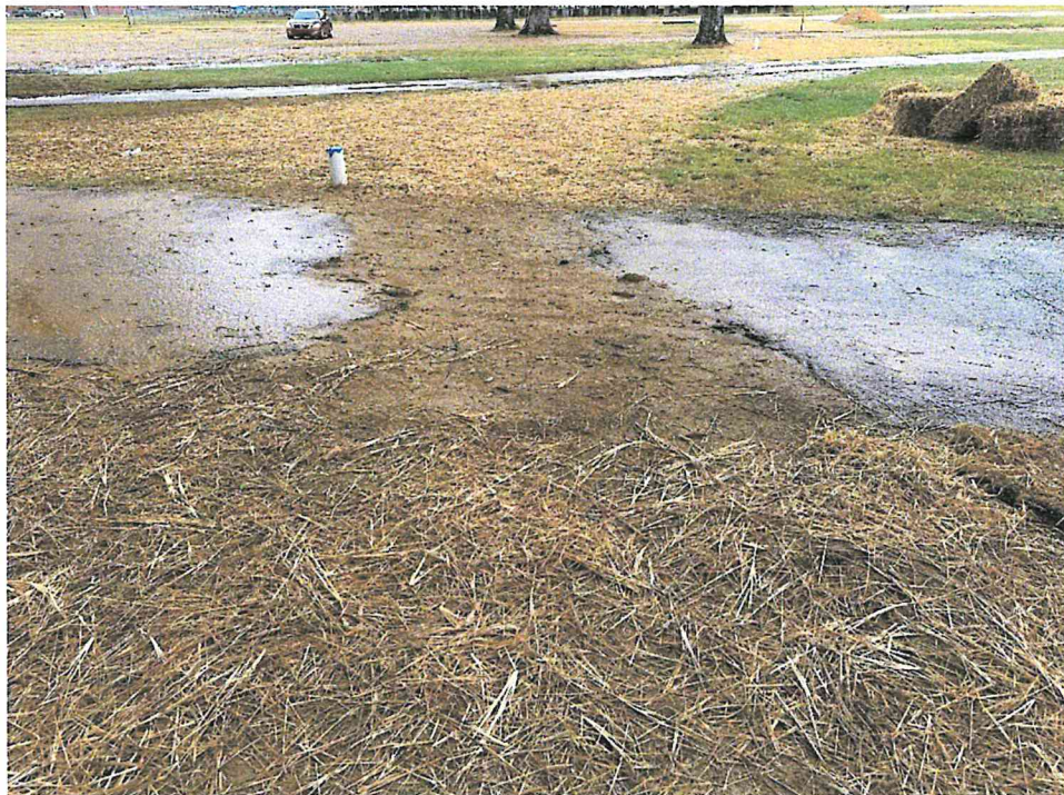
Figure 8 – Repair damaged track where new piping was laid.
